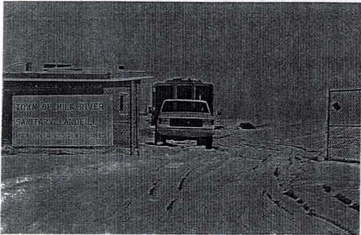
ENTRANCE GATE WITH LANDFILL BUILDING
